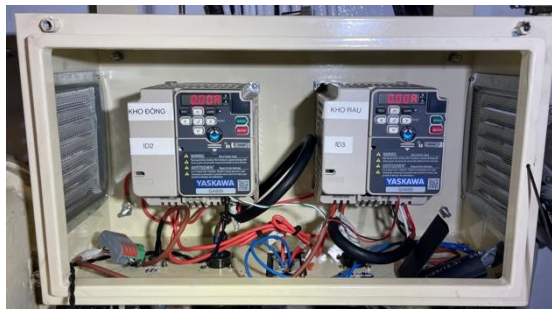
Fig. 5. VFD Cabinet
