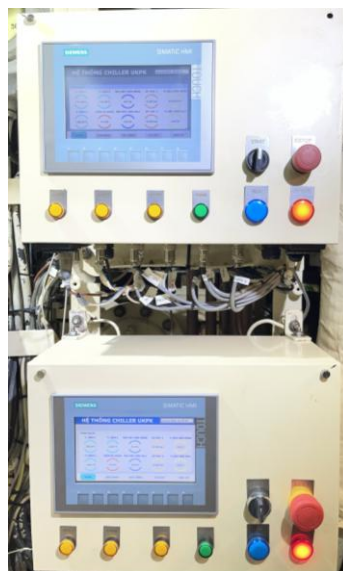
Fig. 6. Dual Control Panels
